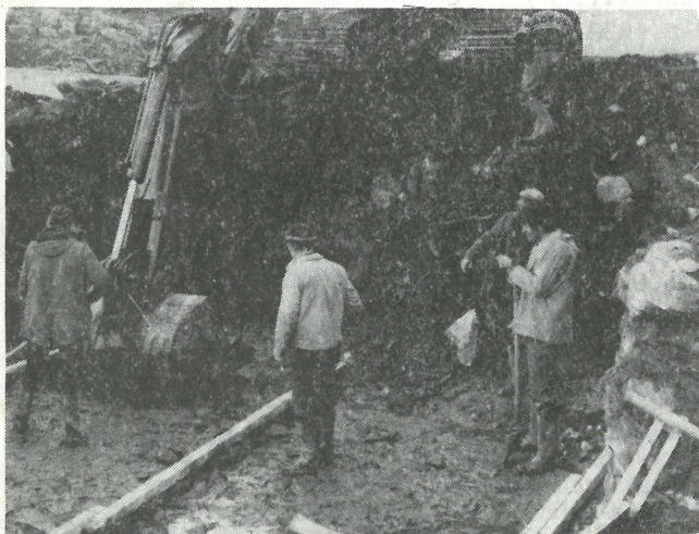
Work in progress on the construction of the Leitir water scheme.
