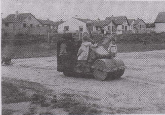
WORK IN PROGRESS IN BALLYBOE.
