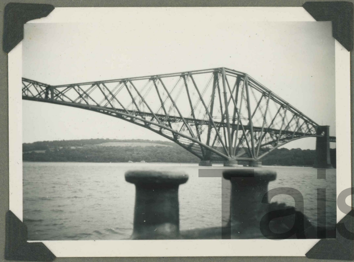
FORTH BRIDGE FROM A QUEENSFERRY BOAT.
