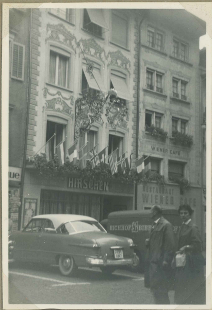
PAINTED HOUSE FRONT IN OLD LUCERNE (WEGGIS- GASSE).
