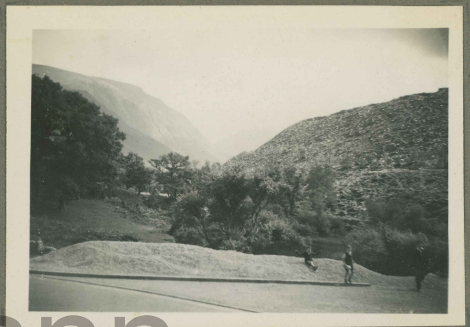
VIEW FROM A5 NEAR BETHESDA LOOKING S. WITH A SLATE- QUARRY ON THE RIGHT.
