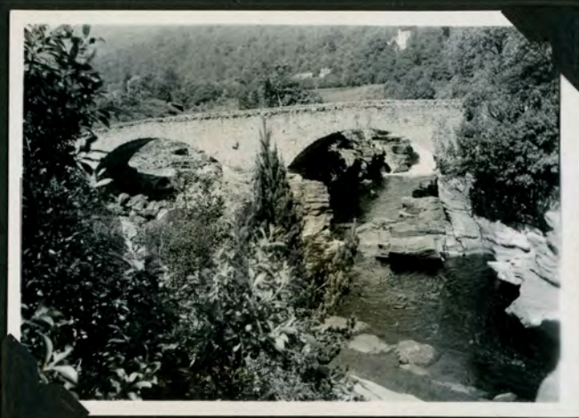
OLD BRIDGE OVER RIVER MORISTON, AT INVERMORISTON.
