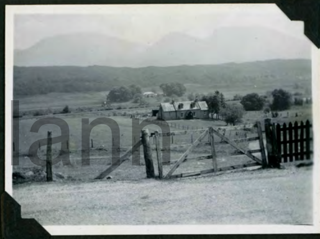
NEAR SPEAN BRIDGE, NORTH SIDE.
