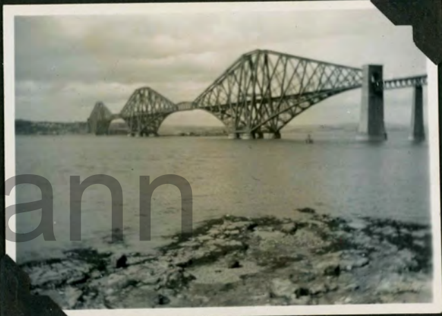
FORTH BRIDGE. QUEENSFERRY. MIDLOTHIAN
