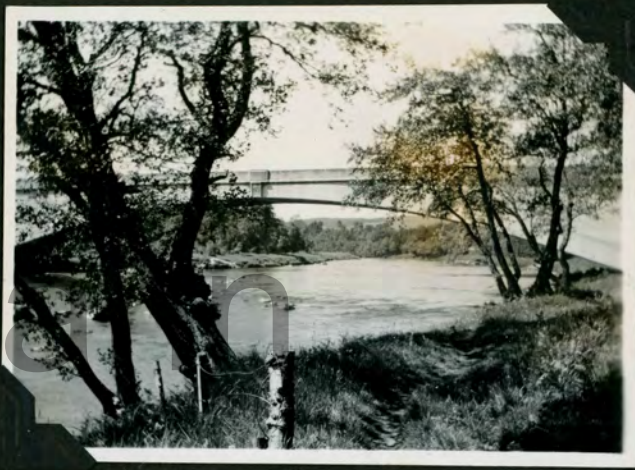
SPEY BRIDGE, OVER THE RIVER STRATH NEAR GRANTOWN, MORAYSHIRE.
