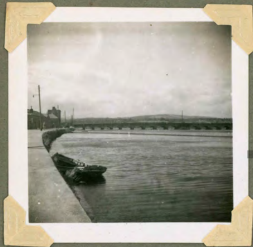
THE BRIDGE INTO ARKLOW.
